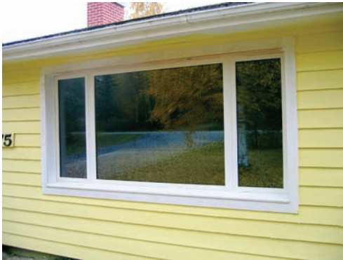
Figure 5. A finished view of the "superwindow" in Sept. 2005.
